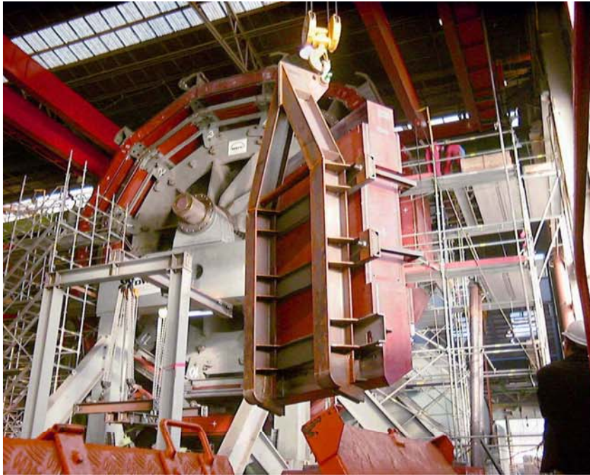
Pre-assembly at Deggendorf (1999)
