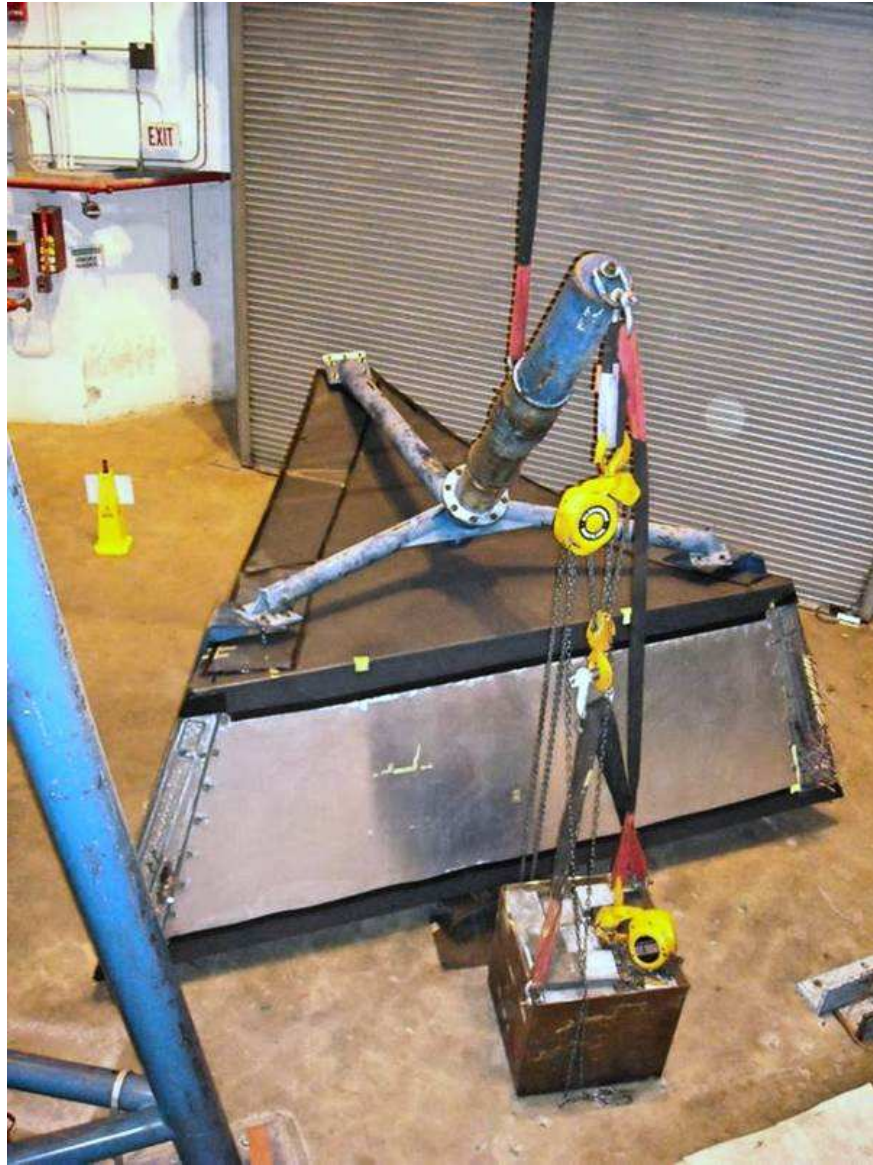
Figure 95: Example of the tools for the installation of one LTCC module that may be used also for the RICH.
